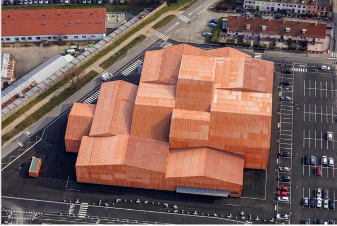
↑ Manuelle Gautrand Architecture, Le Forum sports, associative and events facility, Saint-Louis, France. Photo: Guillaume Guerin
