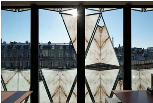
Internal view of the second skin on the front elevation (ph: Manuelle Gautrand)
