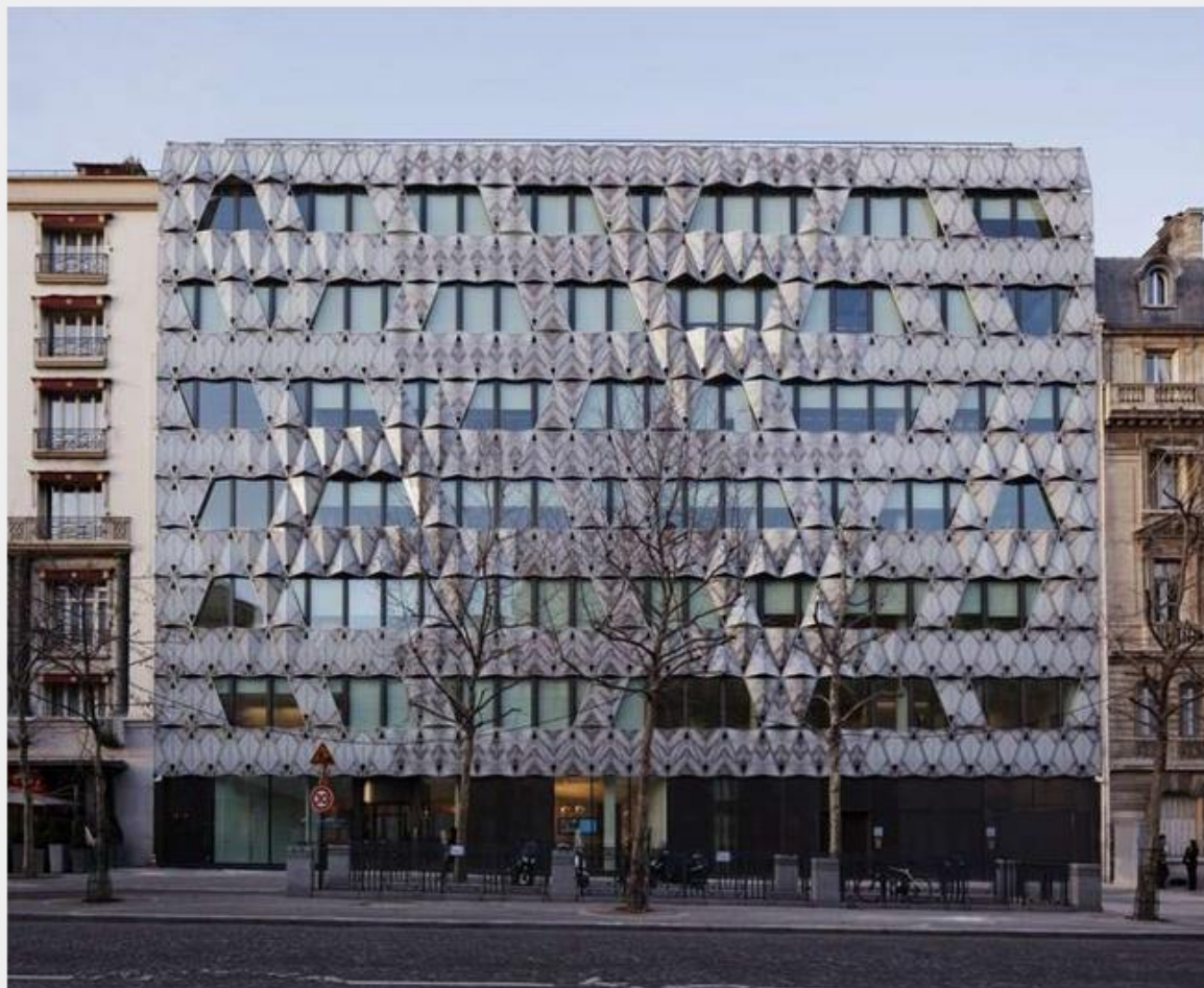
— Office Building Facade
