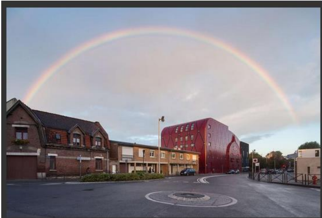
General outside view. Le Palace Theatre 2 by Manuelle Gautrand Architecture. Photography © Luc Boegly. Click above to see larger image.
